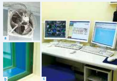
a/ Forced ventilation fan b/ Dual structure window consisting of bulletproof glass and fireproof glass c/ Central monitor room
